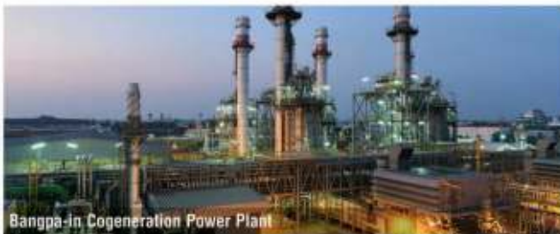
Bangpa-in Cogeneration Power Plant
