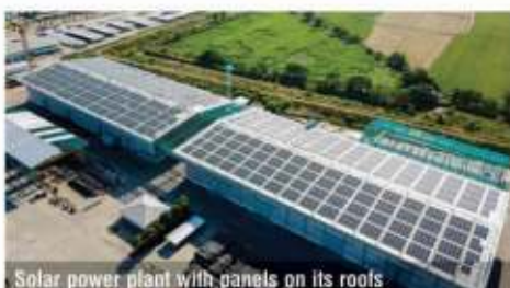
Solar power plant with panels on its roofs
